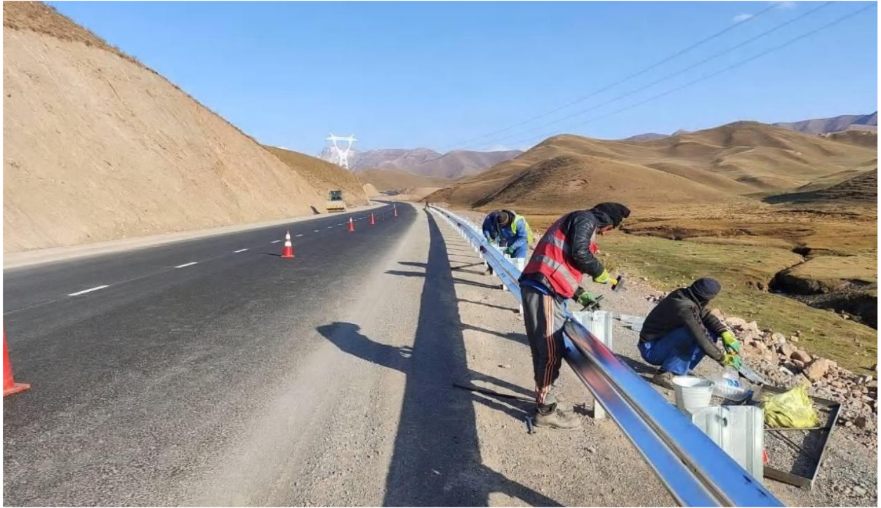
Figure 10: Installation of waveform guardrail, km 113+300 – km 113+512, LHS.
