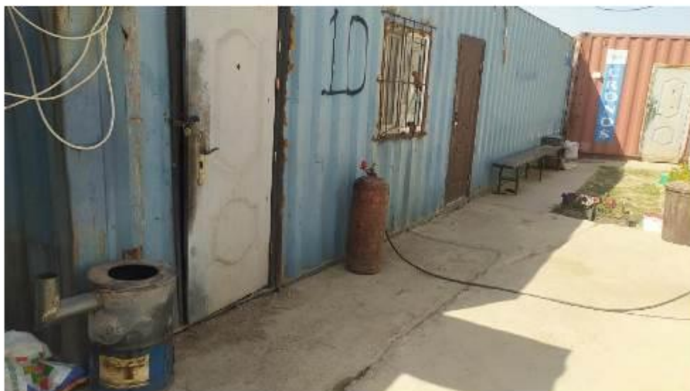
Photo 4. Gas cylinders are still not covered from direct sunlight
