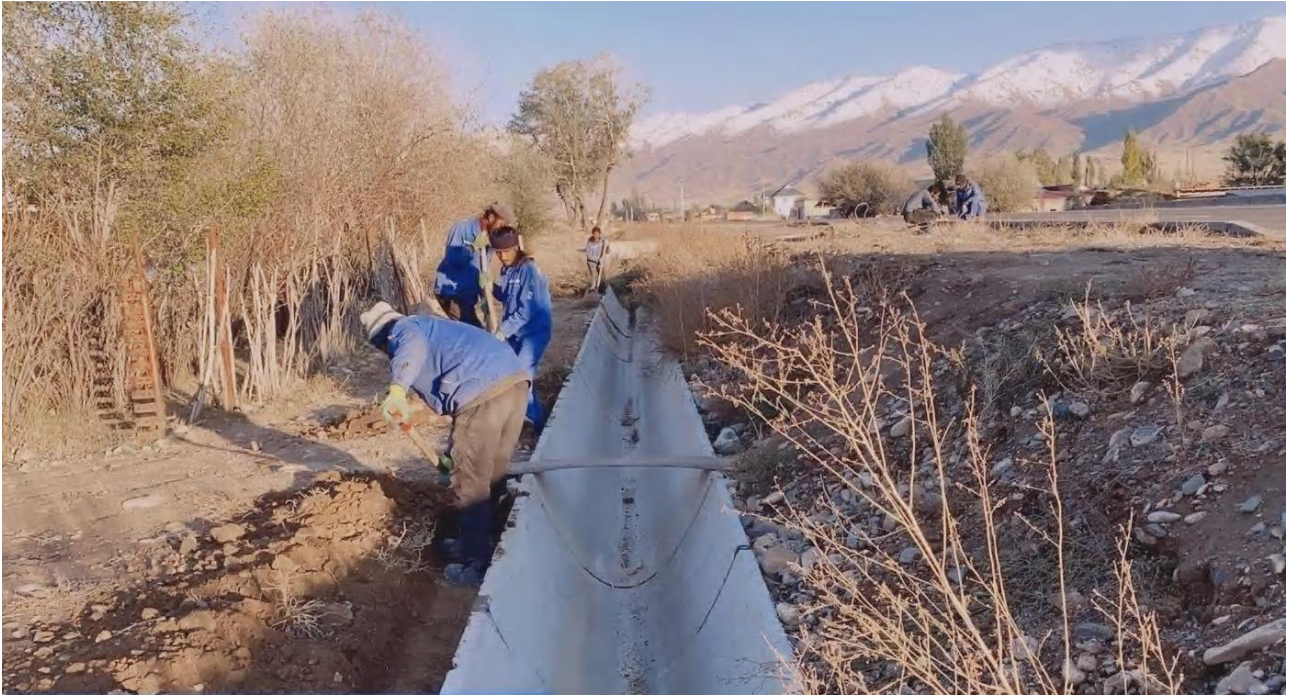
Figure 12: P6 ditch cover plate foundation pouring, km 142+000 RHS.
