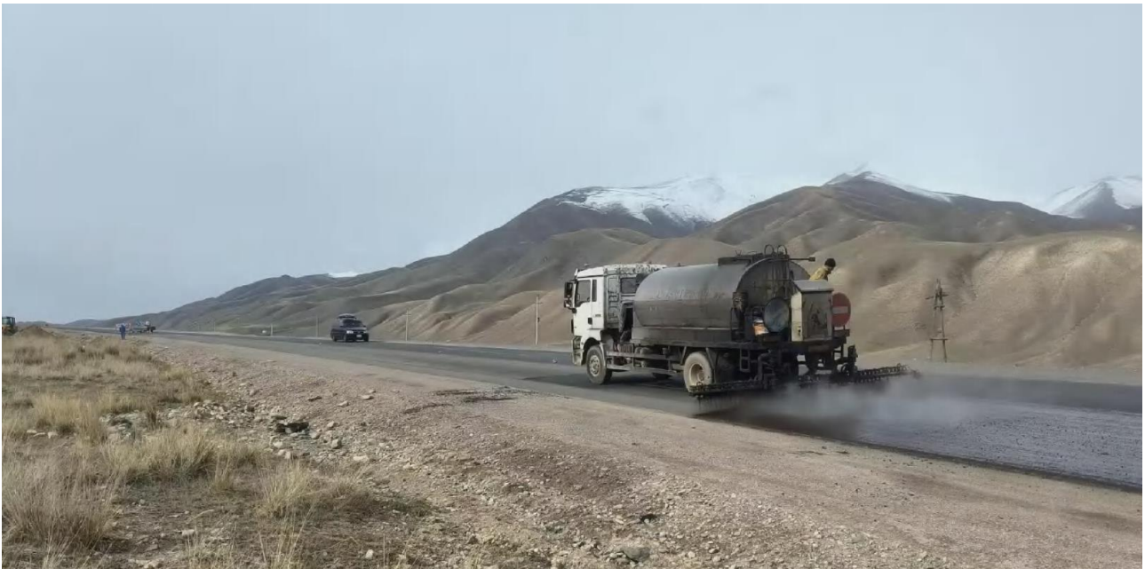
Figure 11: Tack coat, km 102+180 – km 101+120 LHS.
