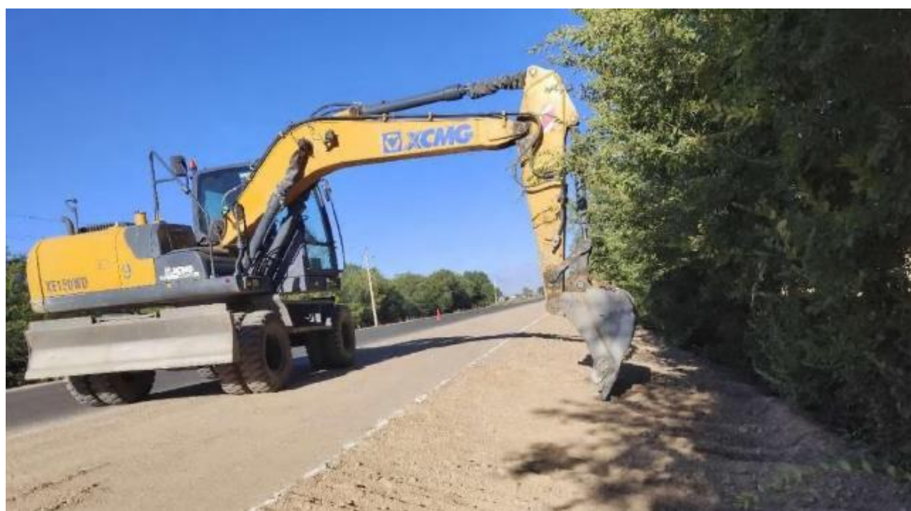
Figure 5: Shoulder slope brushing, km 137+260- km 137+100 RHS.
