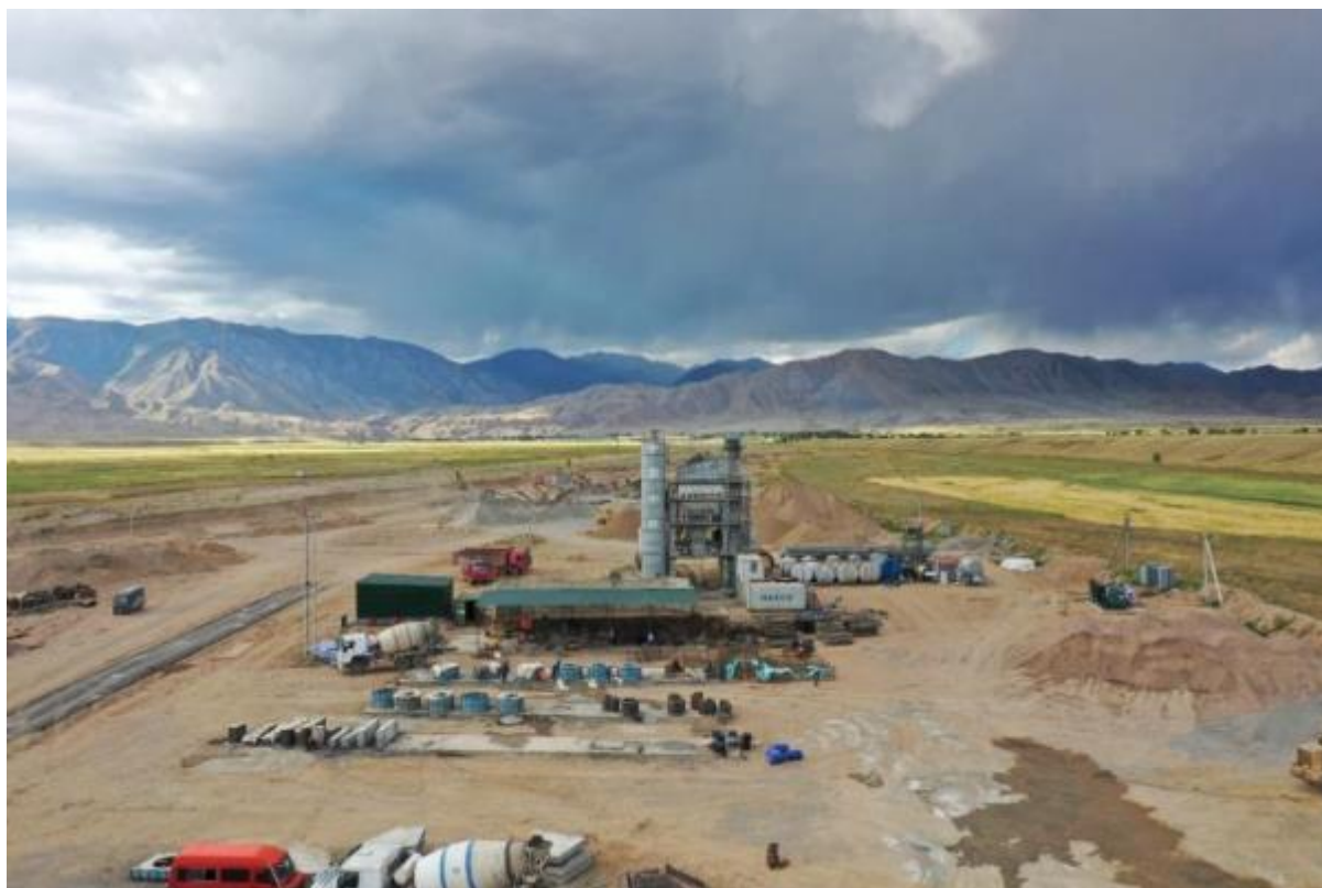
Figure 17: Asphalt plant at the production site (km 148+630).
